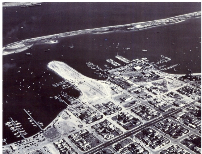
Byron Street mole awaits connection to the rising Shelter Island.
